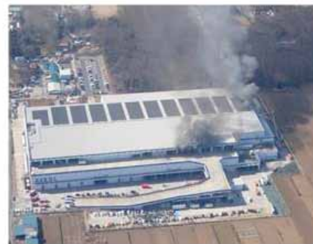
The state of the building at the time of the fire (around 12:00 on February 16) (Provided by Saitama Fire Fighting Disaster Prevention Air Corps)
