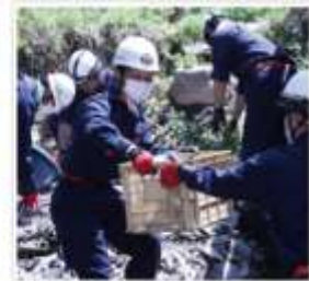
Debris removal (Nishihara Village volunteer fire corps)
