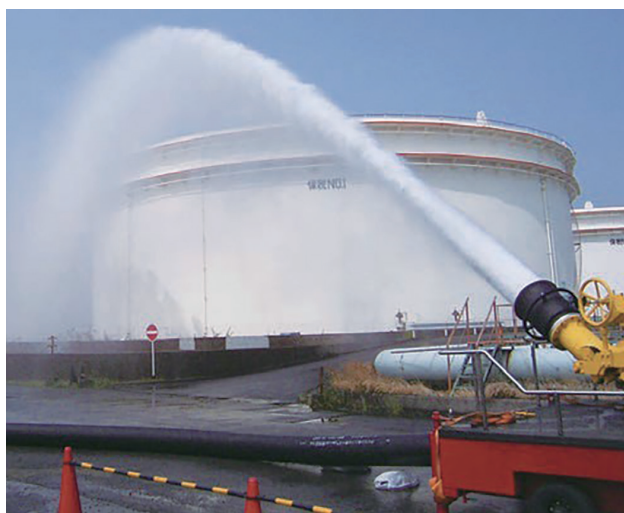
The high capacity foam system
