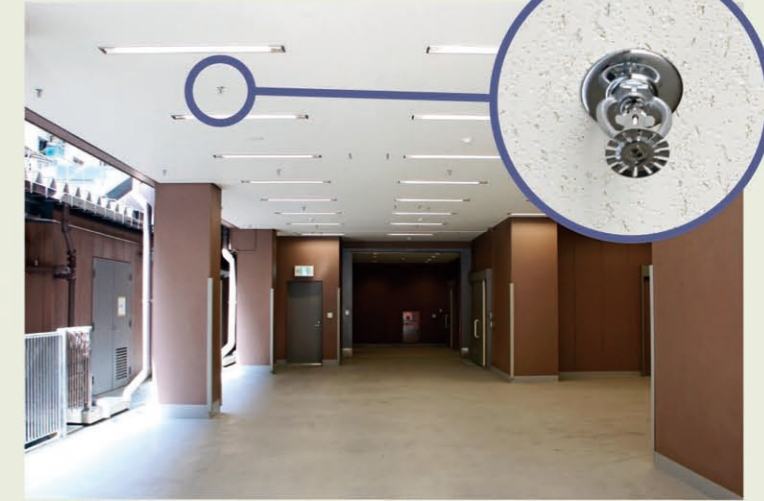
駐車場における閉鎖型水噴霧消火設備 Enclosed water spray extinguishing equipment in parking lots
