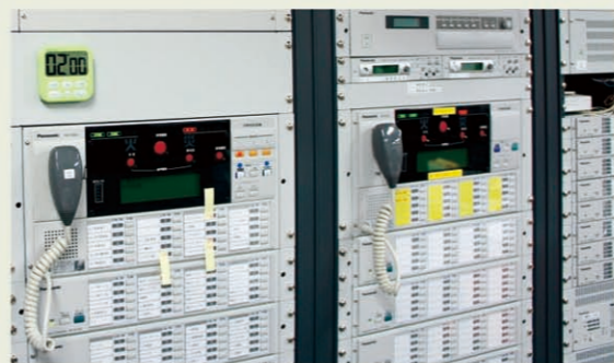
非常警報設備の放送設備 Emergency public address systems for emergency alarm equipment
