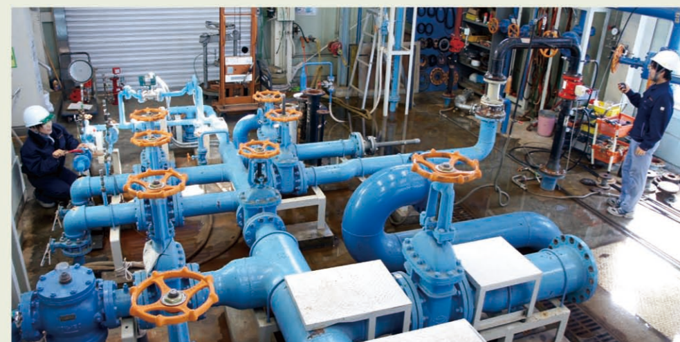
流水検知装置の作動試験 Operating tests of alarm valves
