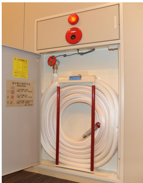
消防用設備等の例（易操作性1号消火栓） Example of fire protection equipment systems (No.1 fire hydrant with easy-operation)
